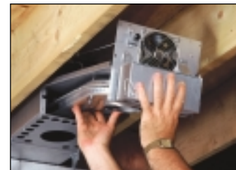
Install Venter Assembly
