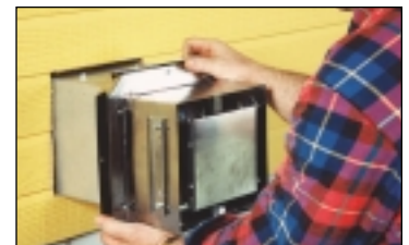
Install Vent Termination
